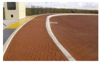
Photo 2 Permeable Clay Pavement
