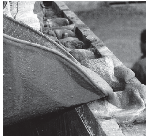
Figure 40 Fluid Grout
